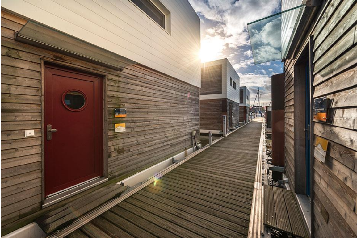
Fortified river banks in inner city areas, ports and former military compounds situated on water are all suitable locations for floating homes
